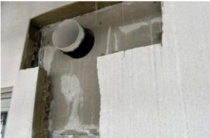
A photo showing Phase 2 North Elevation – EWI removal works around existing vent ducts complete.
