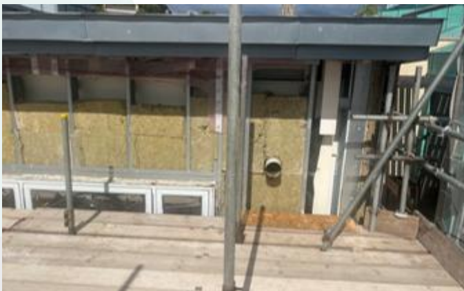
Phase 1 South Elevation
